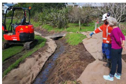
Tysxun Skeen, Downer Construction, discusses the work with MWP's Cathy Brehmer.
