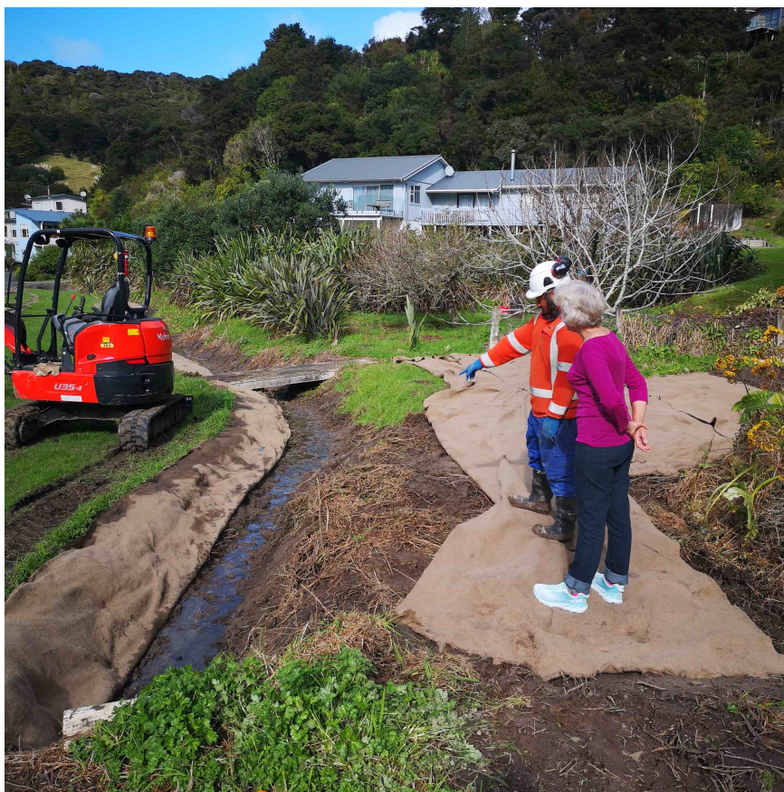
A Downer Construction employee discusses the work with MWP's Cathy Brehmer.
